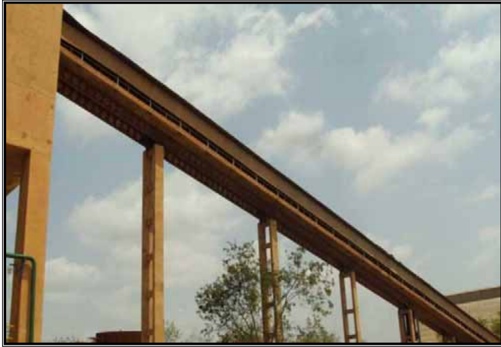
(B) Crusher to Raw mill “ Covered belt conveyor”
