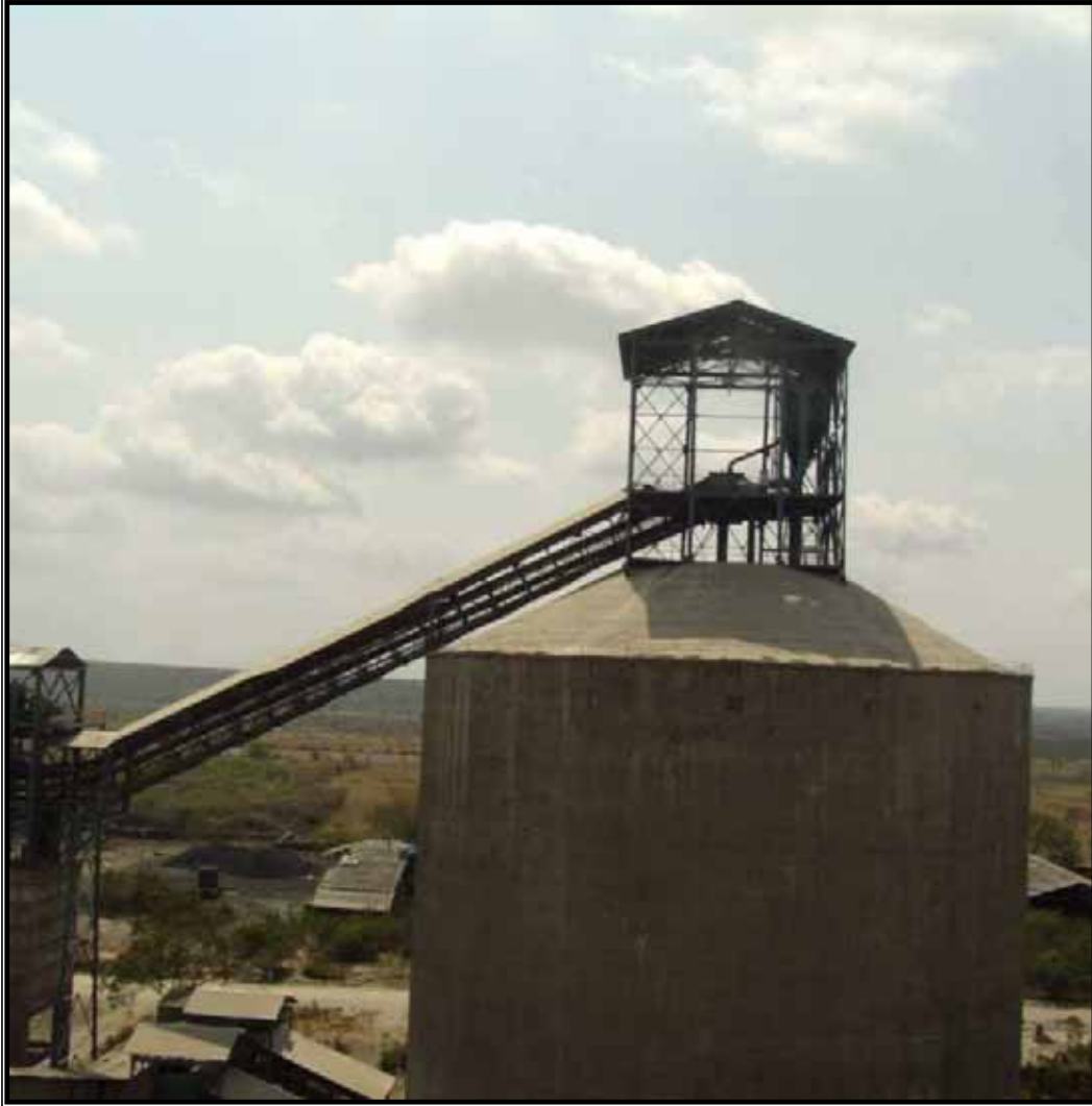
(D) Clinker silo with covered conveyor and Bag filter
