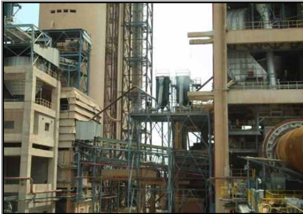
(C) Bag filters installed at transfer points
